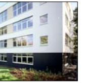
Insulated render and panels between windows
