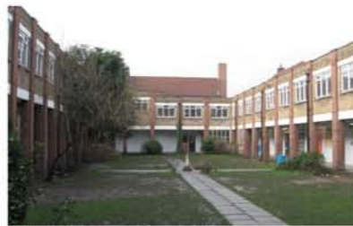
2 View from existing building
